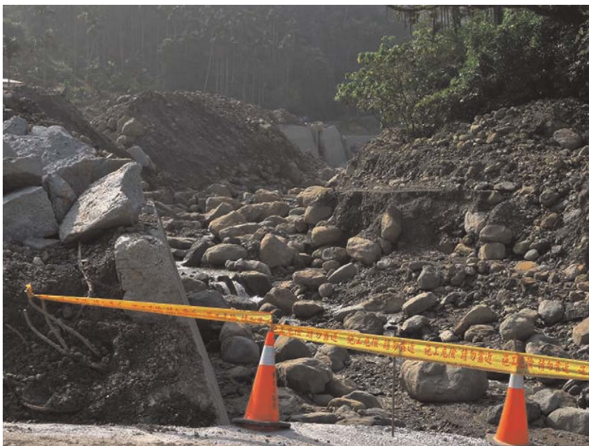
Fig. 4. Debris Flow Occurred in Chayi County During Typhoon Morakot (Photograph Taken by Tsai Mu-Fan).
